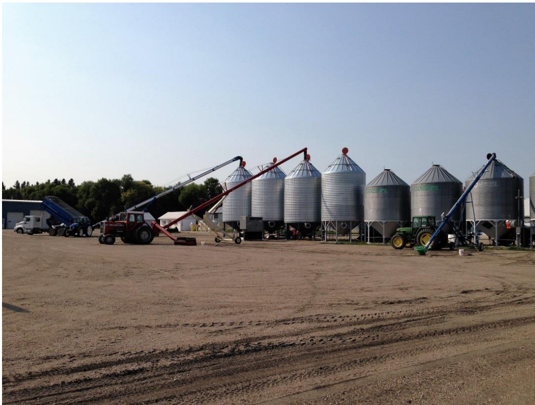
Figure 2: Simultaneous filling of test bins, 2015.
